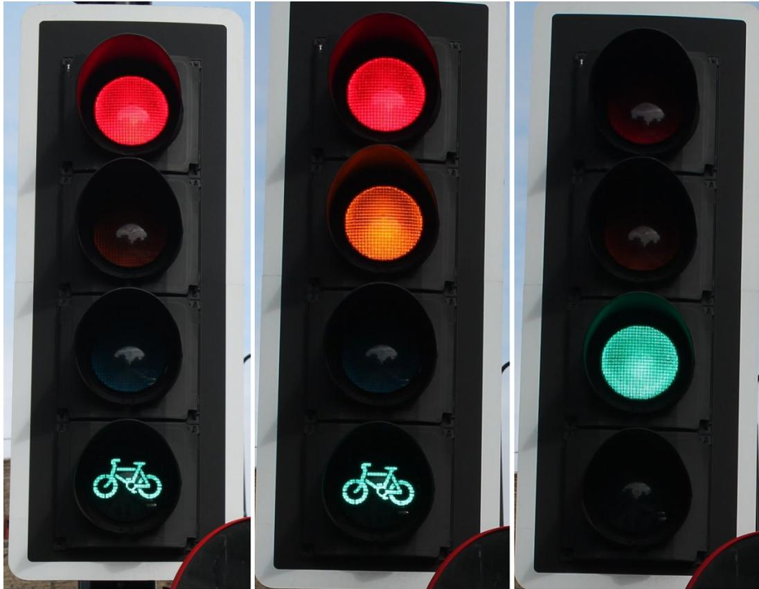
*Figure 2 - Advanced Green Cycle Filter - Appearance & Termination*
