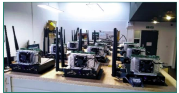
Figure 4: The test bench included 14 sensors, a Siemens controller with a modified configuration (not pictured) and the VIU installed in the same cabinet
